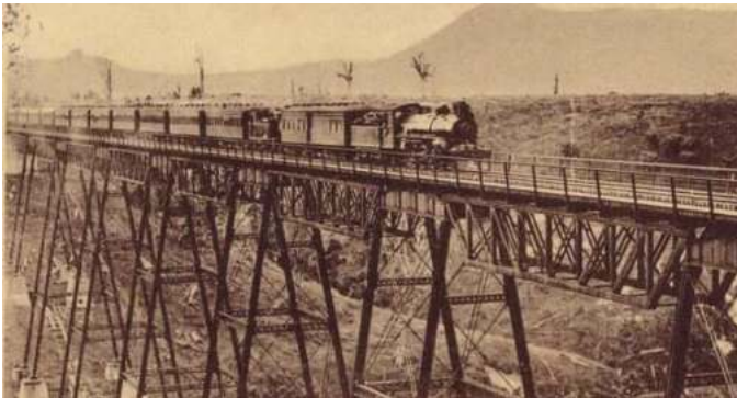
Main Trunk Express on Mangazweka Viaduct.
