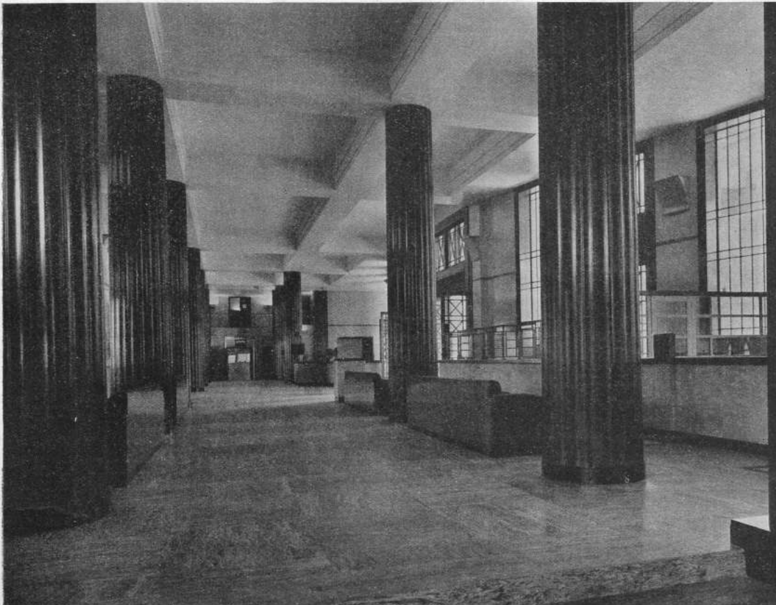
Above, the booking hall: the entrance doors are on the right. This space has been planned to give easy control of large numbers of passengers at one time. The hall is 20 ft. high and has a mezzanine gallery. The panelling in the hall is in Canadian figured birch with horizontal bands of African Zebrano. Architraves and door surrounds are in Burmese teak. The fluted columns, 3 ft. in diameter are also in teak with ebonised bases. The floors of the booking hall and upper floors are of rubber.
